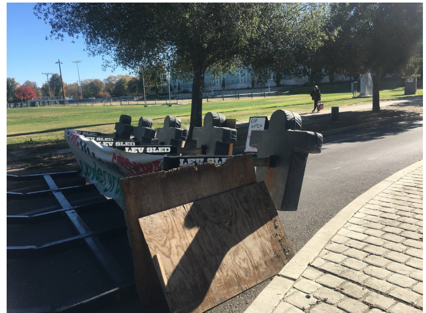
Barricade supported with football blocking sleds
